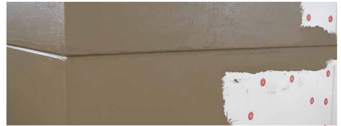
First coat of Raso Top 800 skim plaster
